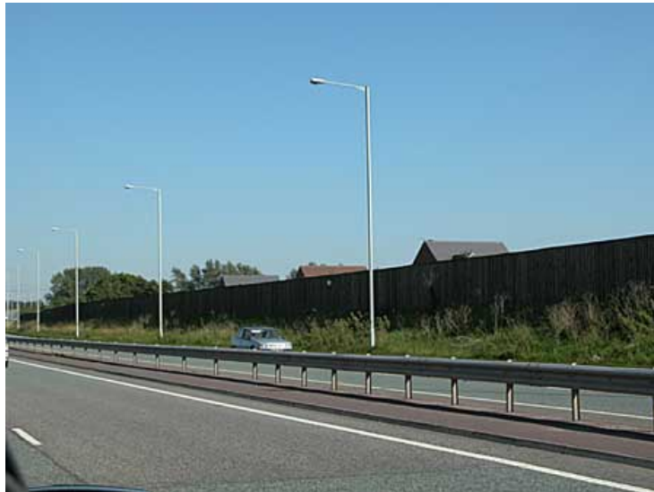
Figure MC1 Example of noise fencing
