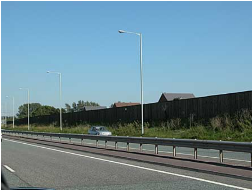
Figure MC6 Example of noise fencing
