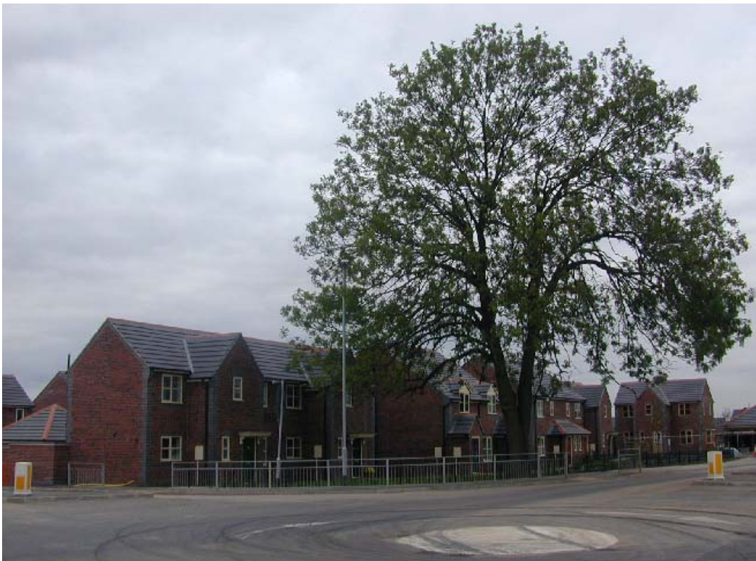
Figure RT1 Retained mature tree showing signs of stress and damage because it is too close to new dwellings and could lead to incompatibility problems in the future
