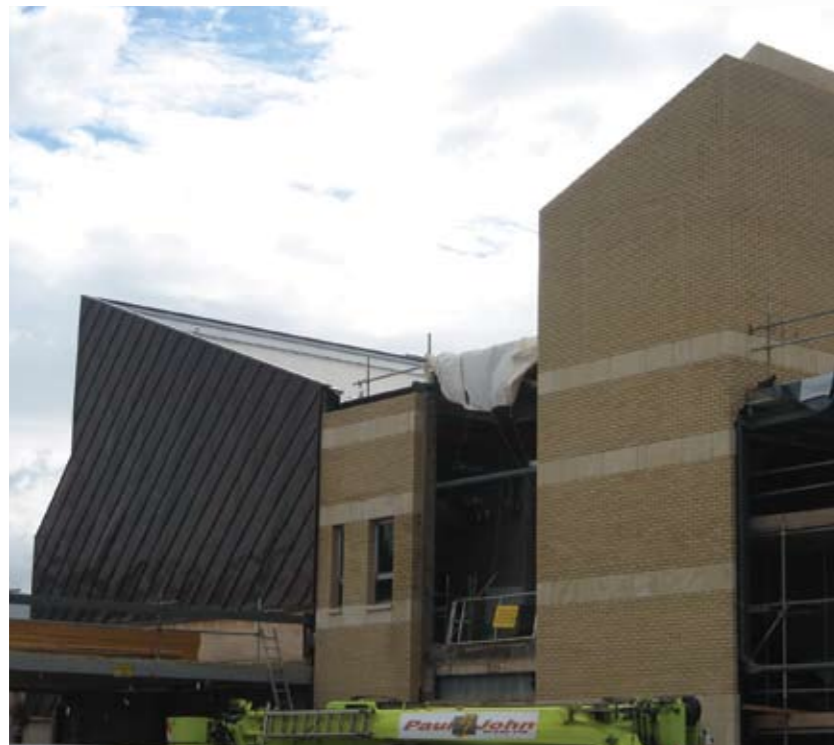
New Magistrates Court Under Construction
