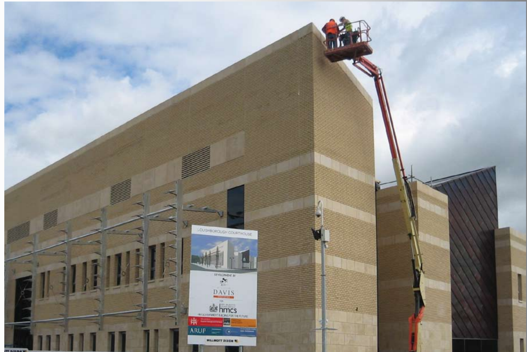
New Magistrates Court Under Construction
